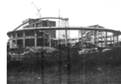
Original Palmer Auditorium under construction.
