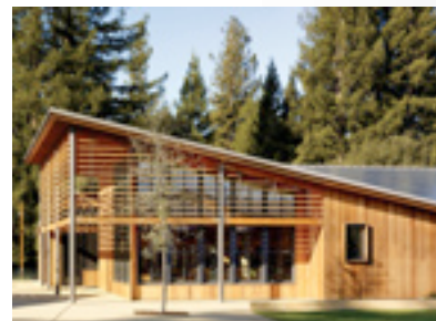
New library building with salvaged redwood siding and Alaskan Yellow Cedar sunscreen louvers.
