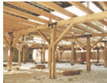
Douglas Fir from St. Lawrence River were reused as columns and beams in the Ottawa store.
