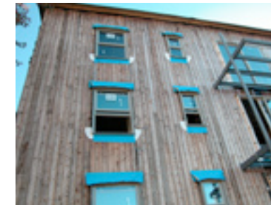
Reclaimed wood forms part of exterior wall assembly.
