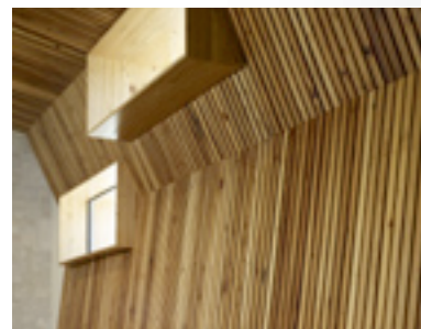
Reclaimed Cypress was used for interior wall and ceiling paneling, as well as library shelving.
