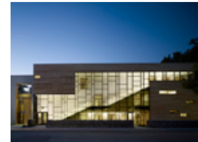
The Jewish Reconstructionist Congregation used reclaimed materials extensively as part of the first LEED Platinum house of worship.
