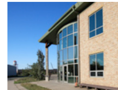
Facade features brick from a deconstructed industrial warehouse.
