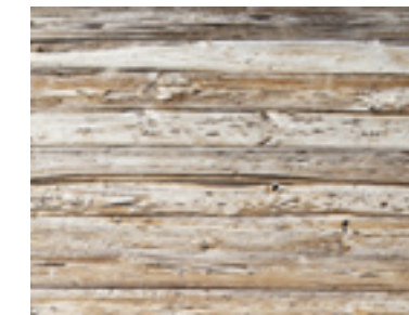
Exterior siding detail.
