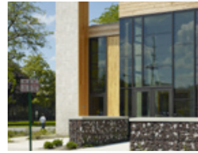
Gabion walls were filled with broken brick from demolition.
